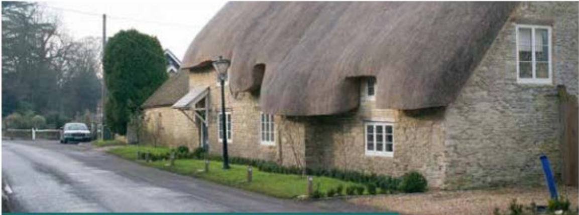
Figure 12: Example of building frontage set directly against public grass verge.
