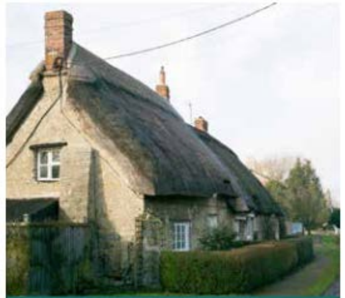
Figure 13: Small landmarks or 'marker' buildings are created where gables front the street (Bramble cottage)
