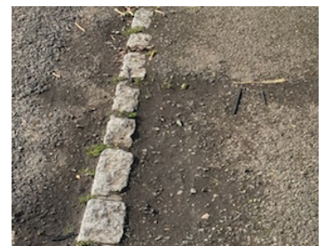
Kerb to footway of granite setts
