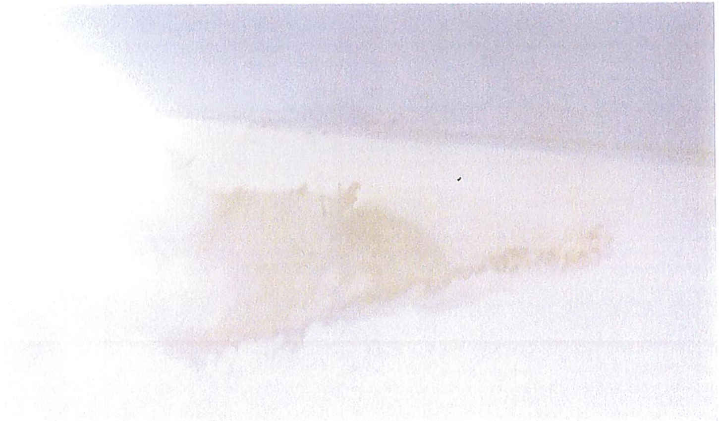
Photo 6: Apparent moisture staining on the perimeter wall of the stairwell.
