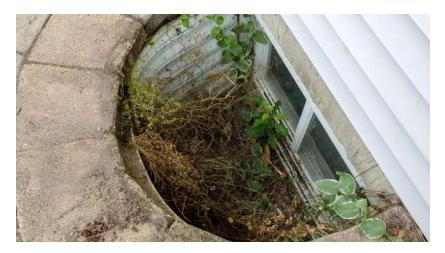
Water and debris can get trapped in your window wells, allowing moisture to intrude into your basement. Clear out any debris, and to avoid this in the future, a clear plastic dome can be installed over the window well to keep water and debris out.
