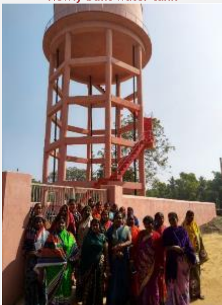
Newly built water tank
