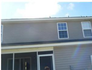
(2) Observed that a section of siding on the screen porch is loose. Recommend notifying the builder so it can be repaired.
