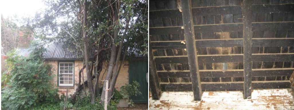
Figures 21 & 22 • Kitchen building (L) and original roof shingles (R) at The Oaks, 2013 • Source: Philip Leeson Architects.
