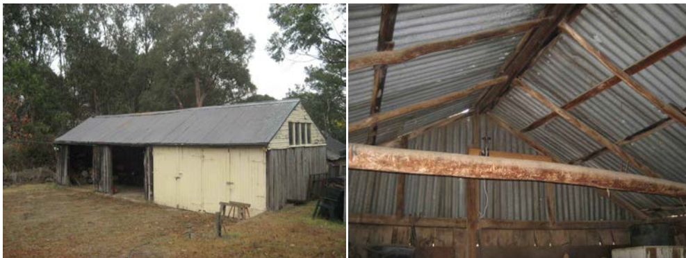
Figure 27 • Reclaimed slab garage (L) and bush pole construction from inside (R) at The Oaks, 2013 • Source: Philip Leeson Architects.
