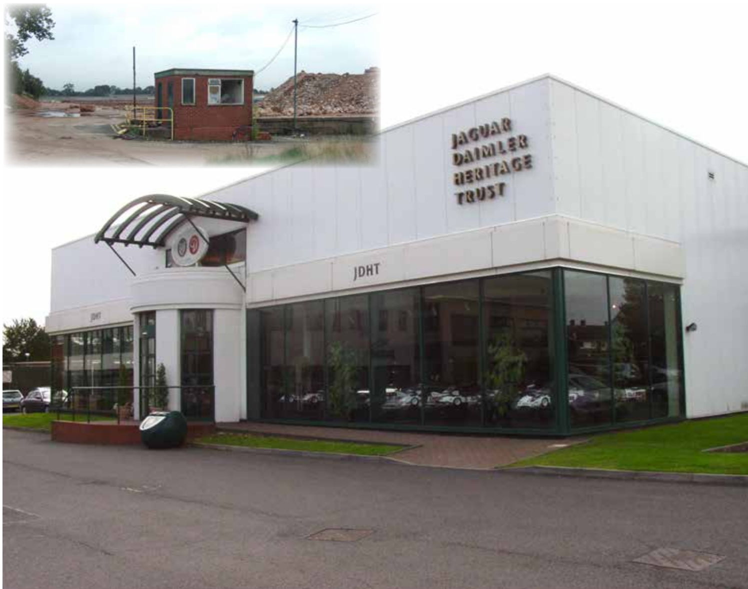
Browns Lane was sold in 2007 and the buildings progressively demolished including the building above. The museum was then moved to two permanent displays in Gaydon and Coventry. The majority of the site was turned into a housing estate known as "Swallow's Nest".
