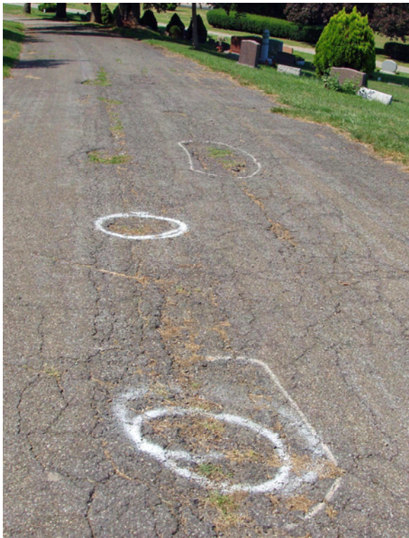
The contractor identified spots of crumbling pavement
