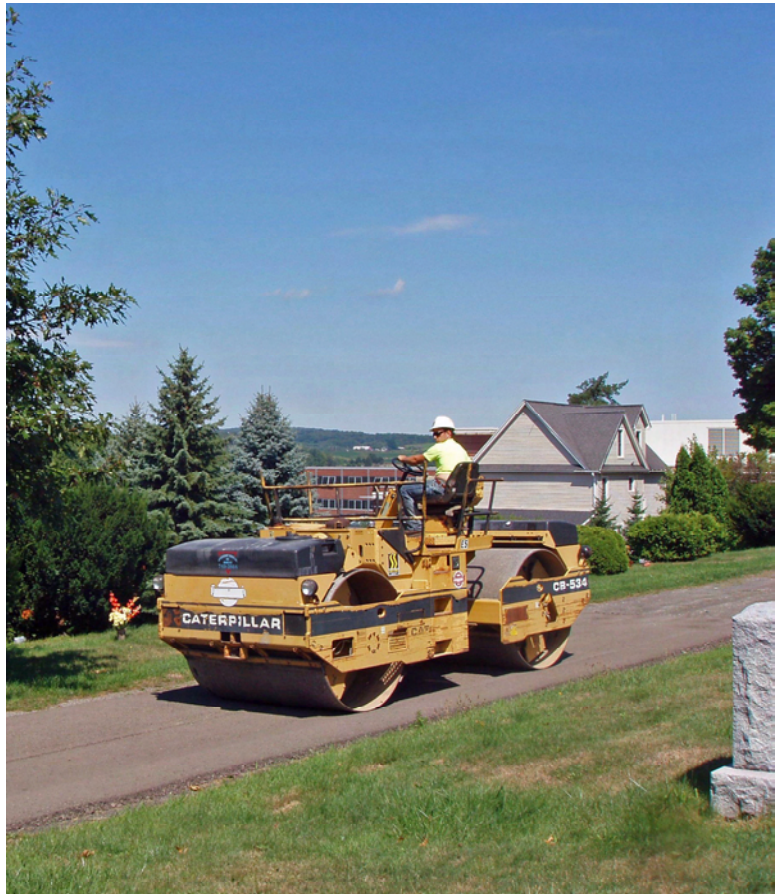
Smoothing the asphalt surface on a perfect summer day, August 2012
