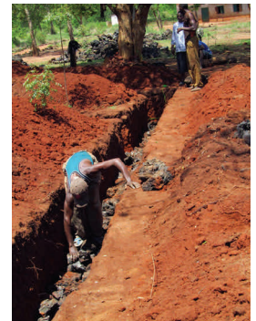
Workers tying rebar and laying rock to be covered with cement for foundation.
