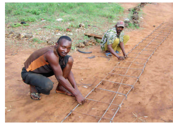
Workers tying rebar and laying rock to be covered with cement for foundation.
