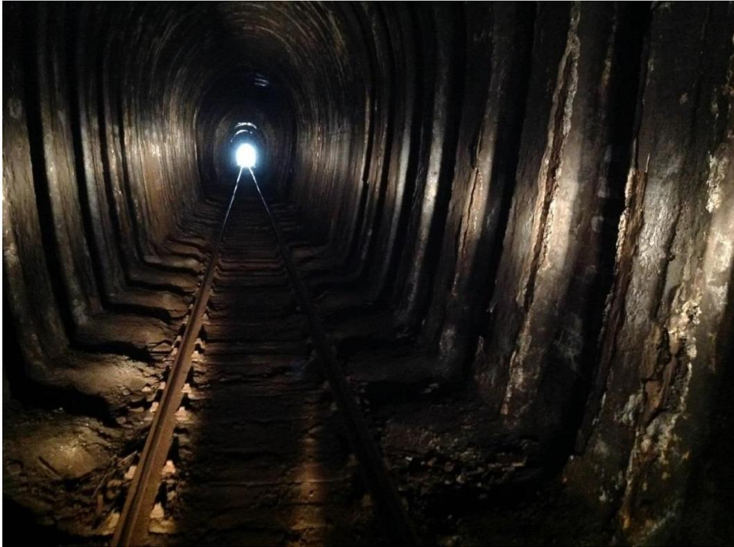
**Figure 33. High-cube container restricted tunnel on the NAL**
