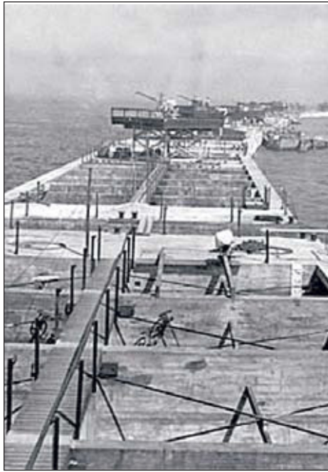
“Mulberry’s” used at beaches during the Normandy Invasion. After serving their initial purpose of getting heavy equipment ashore, they were later ravaged by severe storms along the French coastline and abandoned.
