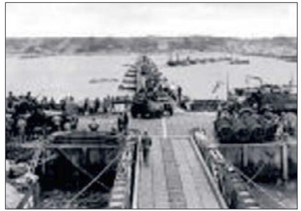
“Mulberry’s” used at beaches during the Normandy Invasion. After serving their initial purpose of getting heavy equipment ashore, they were later ravaged by severe storms along the French coastline and abandoned.
