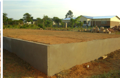
Storage room Construction
