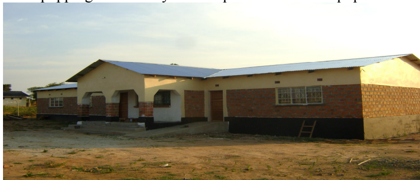
House/Sick bay finished
