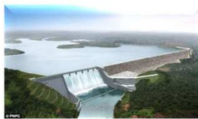
Xe-Pian Xe-Namnoy Hydroelectric Power Project
