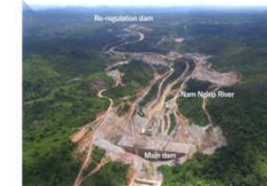
Nam Ngiep Dam Project
