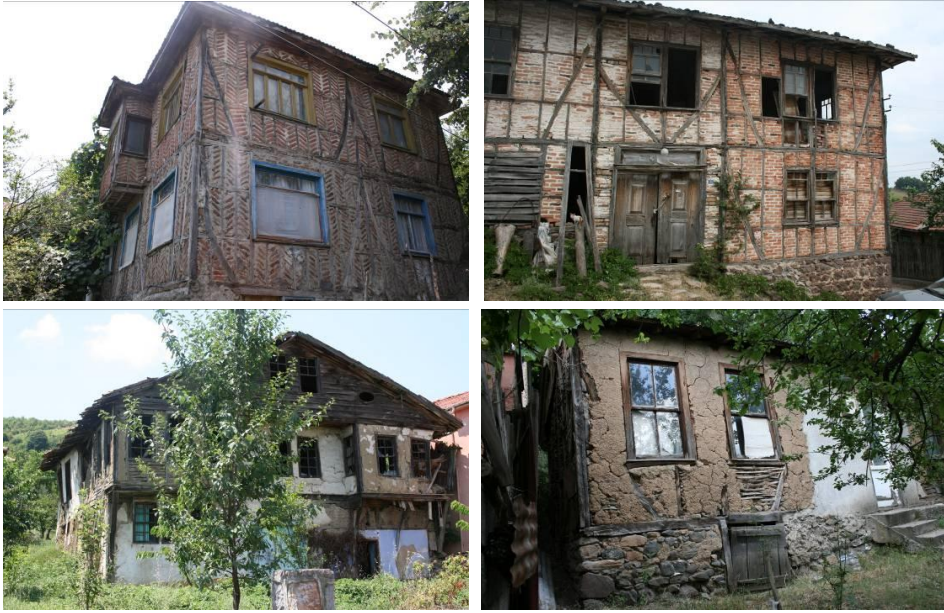
Figure 1: Hımış-style wall with stone infill laid in mud mortar in Saraylı and Orcun villages.
