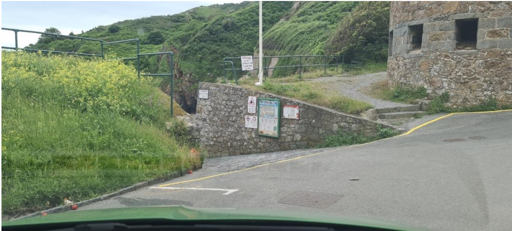
Recticel in front of slipway wall & Martello Tower steps
