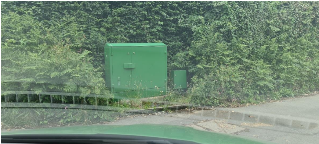
tyres in front of Electric box
