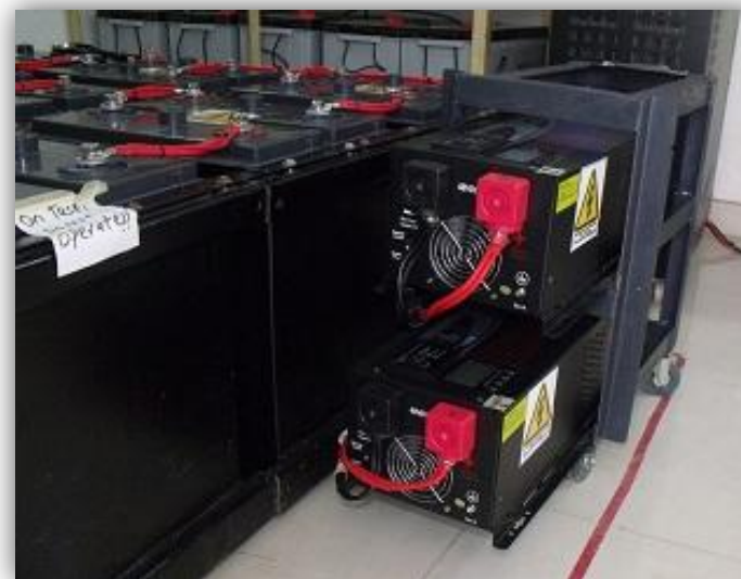
Solar inverter & batter bank
