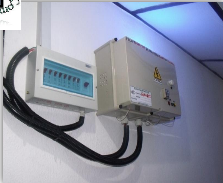
High Powered Appliance Automatic Isolator (AGPOO & PI unit)
