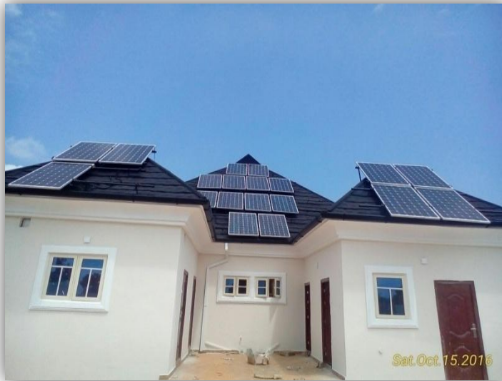
5.0KWp Solar Panel South End Roof
