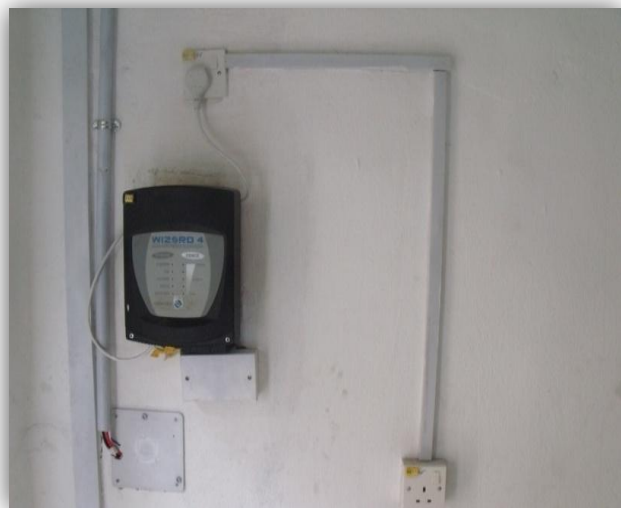
Solar Powered Electric Fence Control Unit
