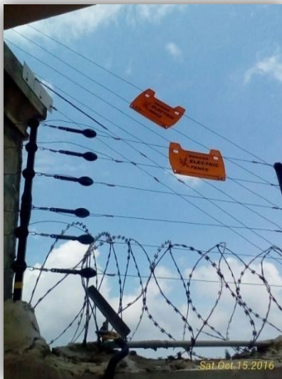
Solar Electric wired fence 12,000Volt high tension
