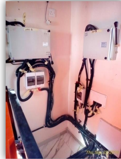
Solar control & safety units in power room
