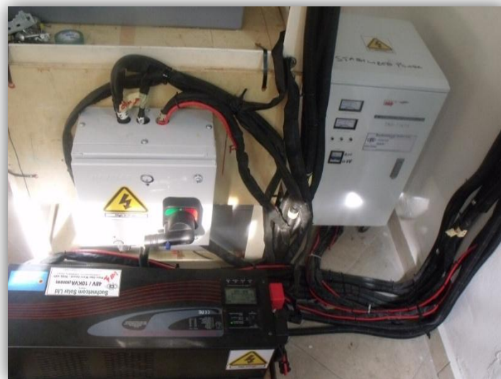
20KVA voltage stabilizer for inverter input
