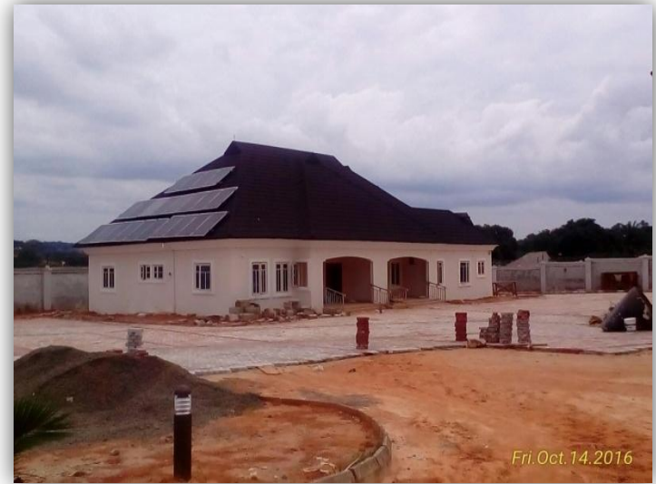
5.5KWp Solar Panel North End Roof
