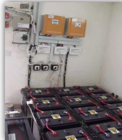
Power Room 20KVA inverter, 72.KWh battery bank
