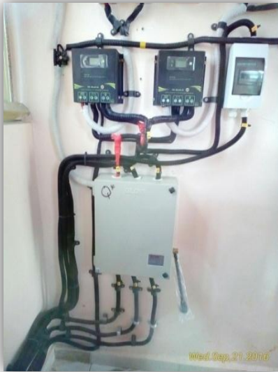
Solar control units in power room
