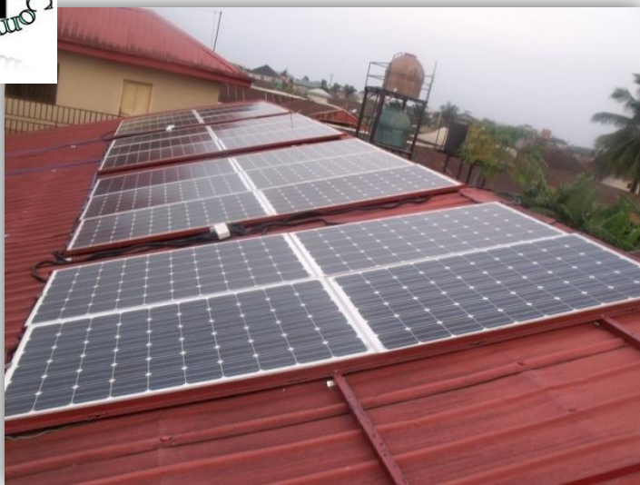
Roof Mount Solar Panel - 6KW
