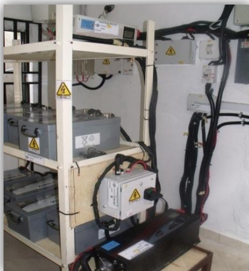
Power Control Room - 11.5KVA Inverter, 25KWh Battery Bank
