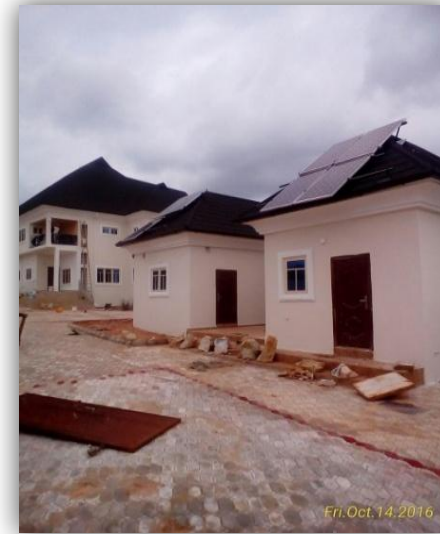
5.0KWp Solar Panel South End Roof
