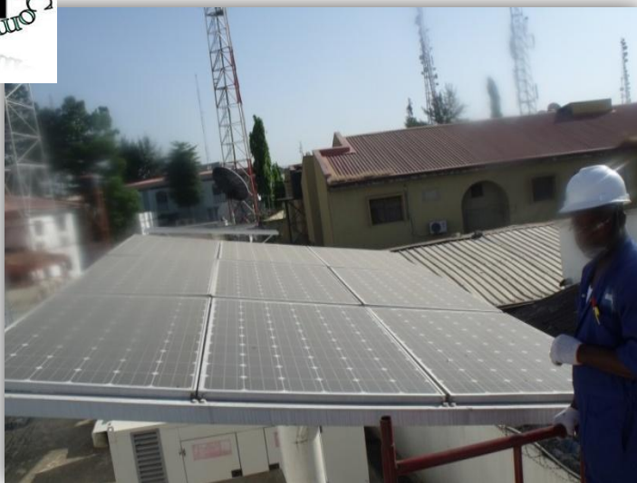
Pole-mount Solar Panel 5.5KW
