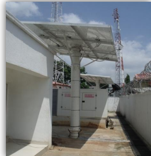
Pole-mount solar panel 5.5KW
