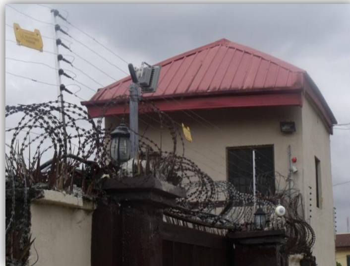
Solar powered electric fence & human presence monitoring sensors
