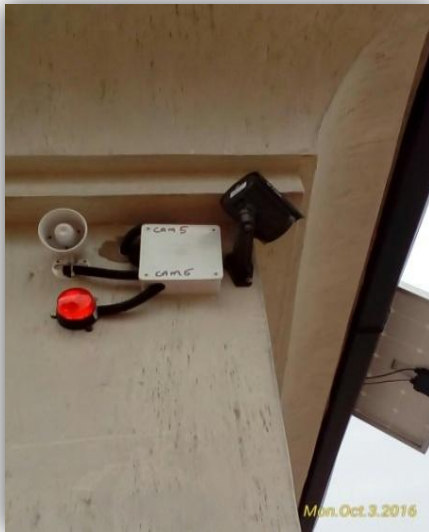
CCTV Surveillance camera, strobe & alarm sounder
