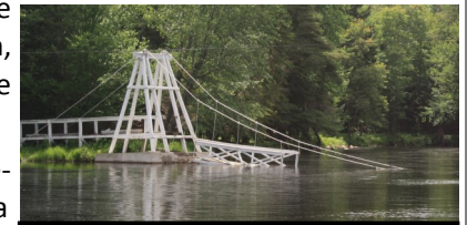
Last pieces of the footbridge as it was dismantled.
