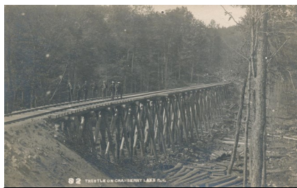
Original 400 ft trestle built for trains to access the Wanakena depot & mills.
