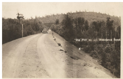
The “Big Fill” used for auto access after rails were removed.
