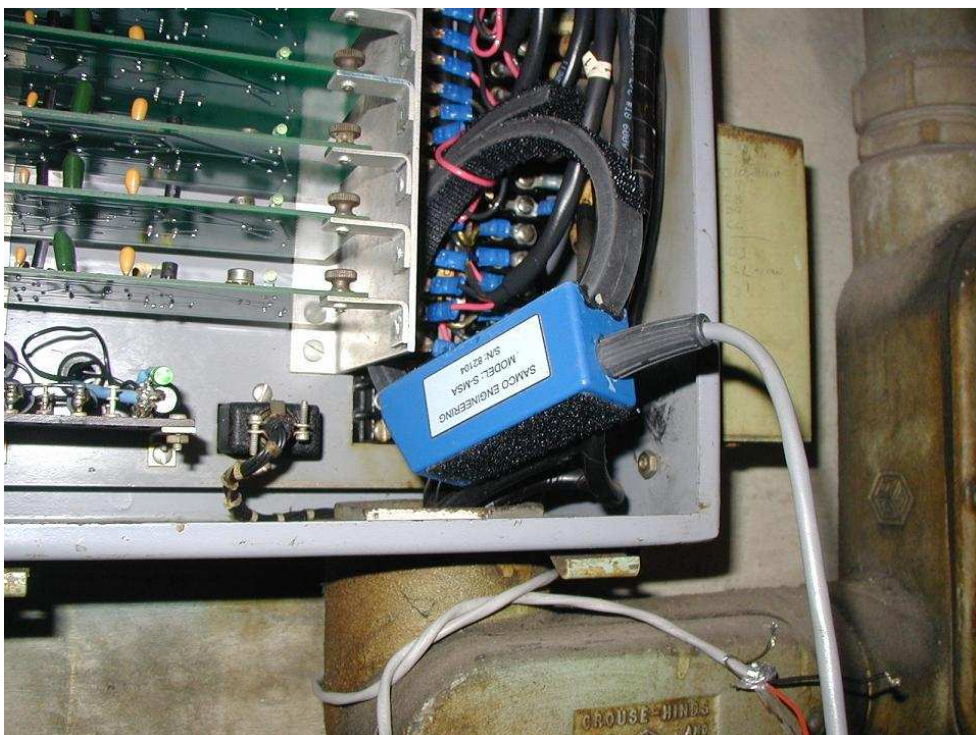
Fig. 4, Small Magnetic Sensor Assembly (S-MSA) around a single conductor
