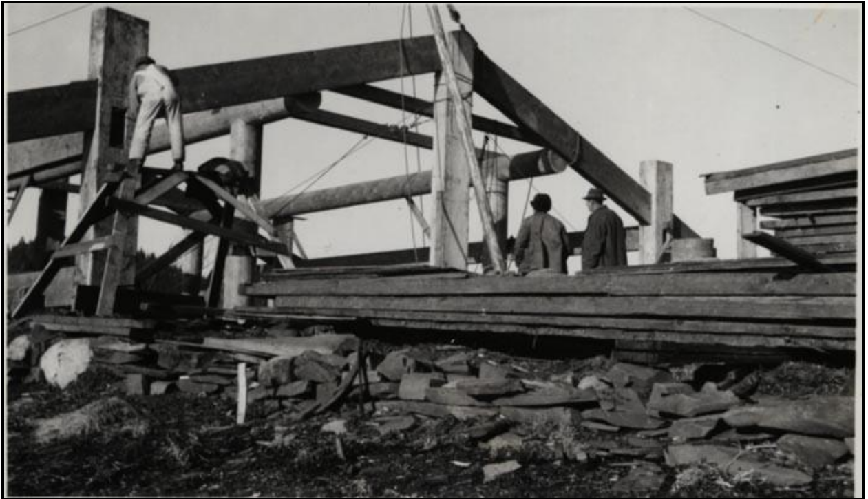
Fig. 49. Construction of Chief Shakes Tribal House, Wrangell, AK. 1940. (Unknown 1940b)
