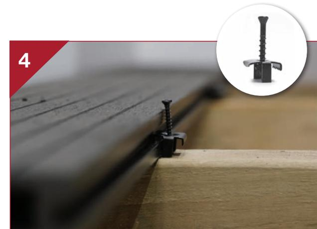
It is very important to install one locking clip per board onto the joist nearest the centre of the board. This helps maintain a consistent expansion gap at the short ends. Failure to use the locking clip will result in uneven gapping at short ends. **Attn: Each board only requires one locking clip in the middle. The teeth should always face the same direction.**
