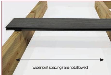
Joists must be set to a maximum of 400mm centres for Portland and Ultrashield Eco (350mm Ultrashield Naturele and Wide Plank). This is to ensure stability and also to avoid warping and cracking of the deck boards.
