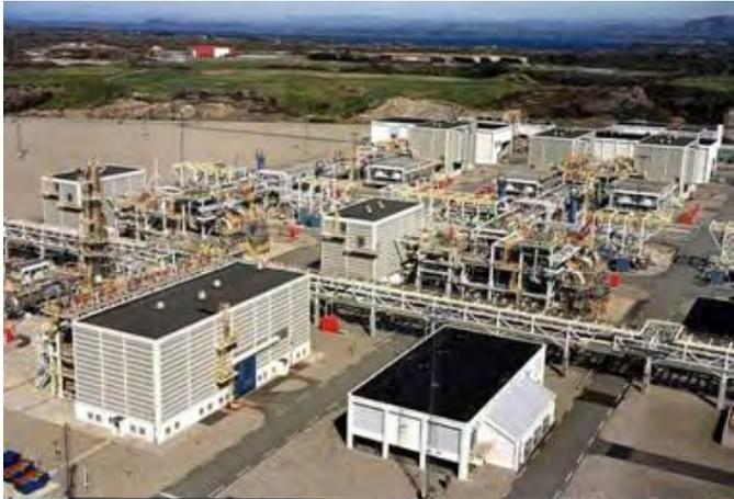
of compression does not require the use of any of the natural gas from the pipe; however it does require a reliable source of electricity nearby. The compression includes a large section of associated equipment such as scrubbers (to remove liquid droplets) and heat exchangers, lube oil treatment etc.
