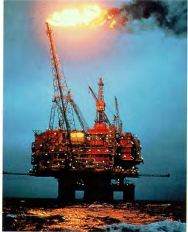
The systems are typically divided into a High Pressure (HP) Flare and a Low Pressure (LP) flare system. The LP system is operated a little above atmospheric pressure to prevent atmospheric gases such as oxygen flowing back into the vent and flare system and generating a combustible mixture. With low gas flow, inert gas is injected at the flare nozzle to prevent air ingress.
