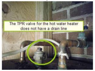
(3) For your reference, the TPR valve is a safety device which is designed to release hot water and steam (and thus relieve pressure) if either the temperature or pressure in the tank gets too high. Without a TPR valve, excessive heat could cause a water heater to explode. The purpose of the discharge/drain pipe is to carry water from the valve to the outside of the home. Without a discharge/drain pipe, hot water could scald the homeowner.
