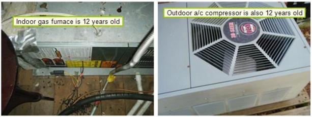
(2) Observed that there is a flexible gas line entering the metal cabinet for the furnace. Instead, there should be a hard pipe which comes out of the cabinet and attaches to the flexible line to ensure the gas line is properly secured. Recommend having an HVAC repairman make the needed repairs.
