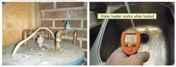
(2) Please note that the TPR (temperature pressure relief) valve does not have a discharge/drain pipe. If this unit is not to be replace in the very near future, recommend having a plumber install a drain pipe which runs down to within 6" of the floor and then extends to the outside of the shed, for safety.
