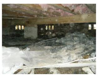
(2) As viewed from inside the crawlspace, observed that there is some standing water in the area under the bathroom. Please note this area is the lowest in the crawlspace and it appears to have come up from the ground and not from the home (i.e. from a leak). To help keep the crawlspace as dry as possible, especially since there is a lot of new wood, recommend having a contractor install a sump pump to reroute excess water to the outside of the home where it can drain away from the foundation.
