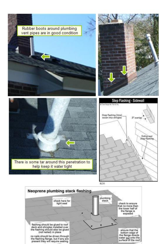
check for buckling or stretching of the flange
