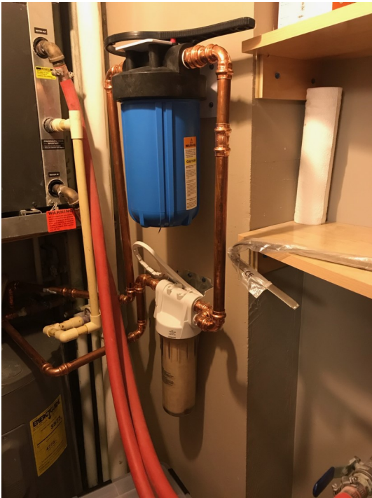
Large Filter is a 5 Micron Charcoal Filter - Color & Odor Small White is 10 Micron Sediment Filter
