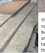
This is known as a baton roll roof ,because of the Belgian roll detail , which are slightly trapesium ( ie tapered) and over which the steel caps are laid
