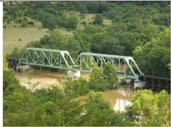
Devil's Elbow rail bridge
