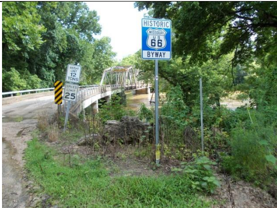
Devil's Elbow Bend Bridge
