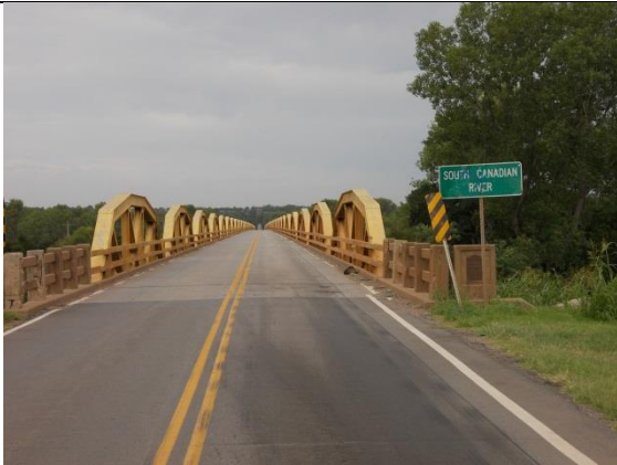
South Canadian River bridge
