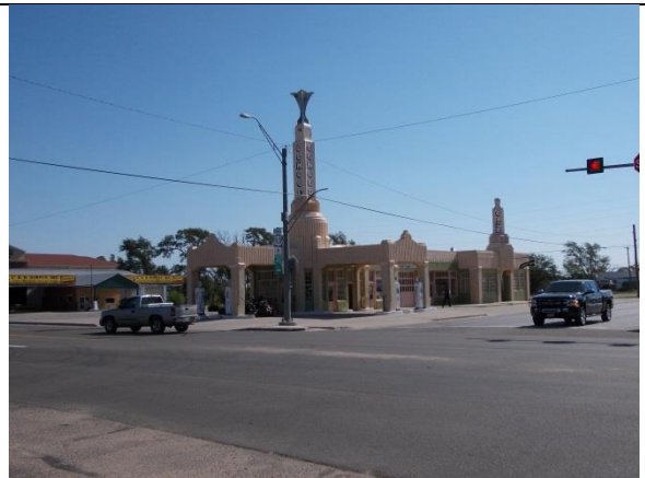
Conoco service station
