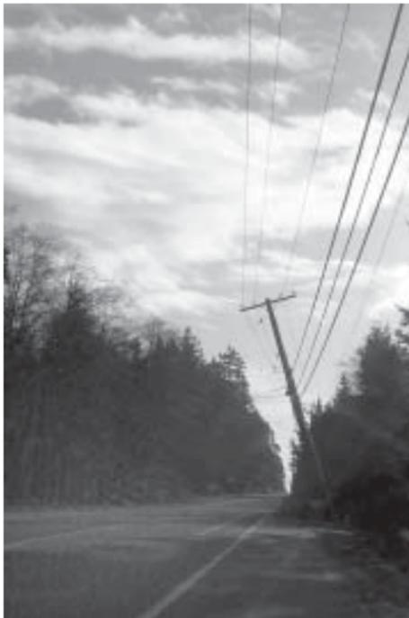
Tired utility pole resting on power lines on the Main Highway. Loop photo
