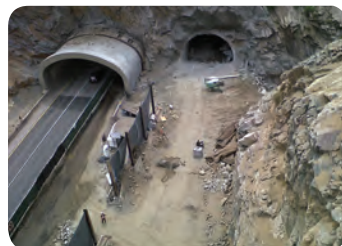
CDOT Twin Tunnels, CO
