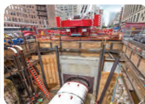
30th Street Rock Tunnel, NYC
