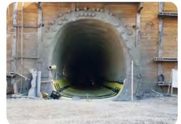
North Temple Square Tunnel, UT
