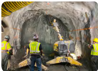
PATH Cross-Passage, NJ
