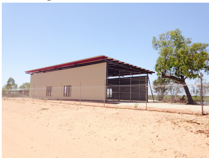
Infrastructure completed in 2014 at Black Rock Landing
