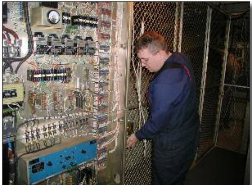
VietnamSeamen Electronics Technician Matt Gross closes a gate on a transmitter at Loran Station Kodiak at Narrow Cape on Kodiak Island. Gross is part of a 7-person crew that keeps the station functioning 24 hours a day, 7 days a week. Photo by PA1 Keith Alholm.
