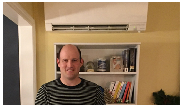
Peter with an indoor wall mounted unit.
