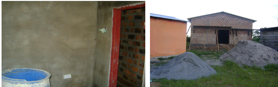
Plastering in progress & materials on site
