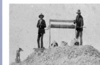
A "Windlass" was one of the first methods of dirt removal from mines. The hand cranked bucket was slow but effective given the resources available at the time.
