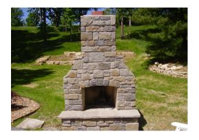
An outdoor fire place is permitted, provided it has an enclosed chamber for combustion as well as a stack or chimney for exhaust. A chamber shall be regarded as enclosed when during the time of combustion, only apertures, ducts, stacks, flues or chimneys necessary to provide combustion air and permit the escape of exhaust gas are open.
