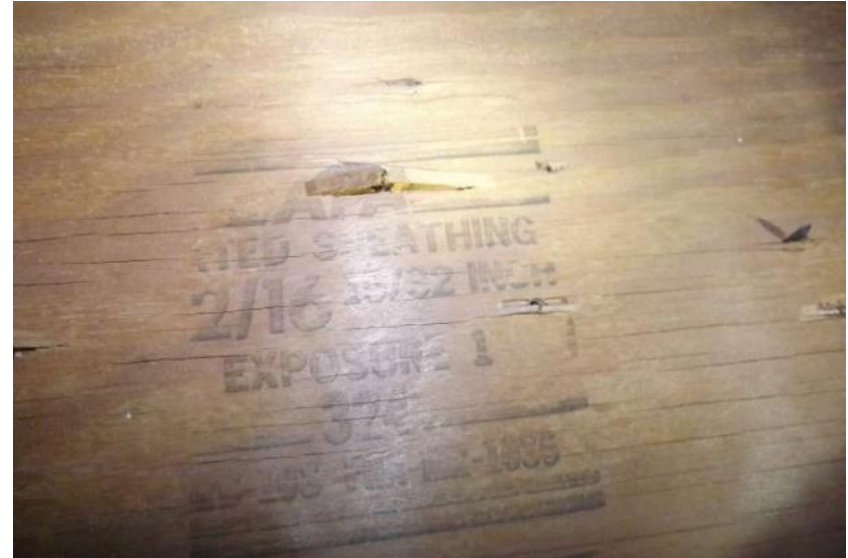
15/32" Deck Thickness Confirmed
