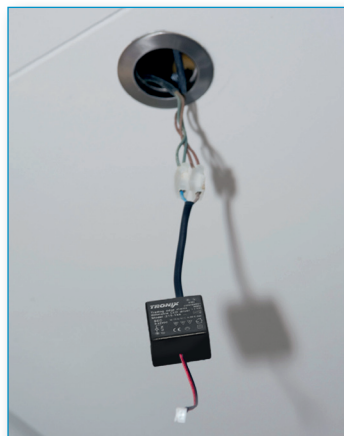
Step 2 Connect the LED driver (215-148) to the terminal block.
