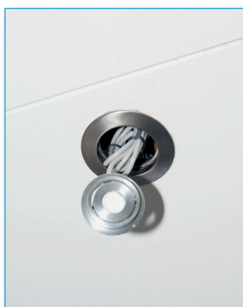
Step 5 Place the LED module back into the fixture.
