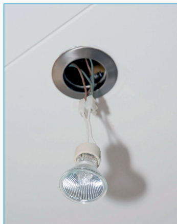
Step 1 Remove the halogen spot from its terminal block.
