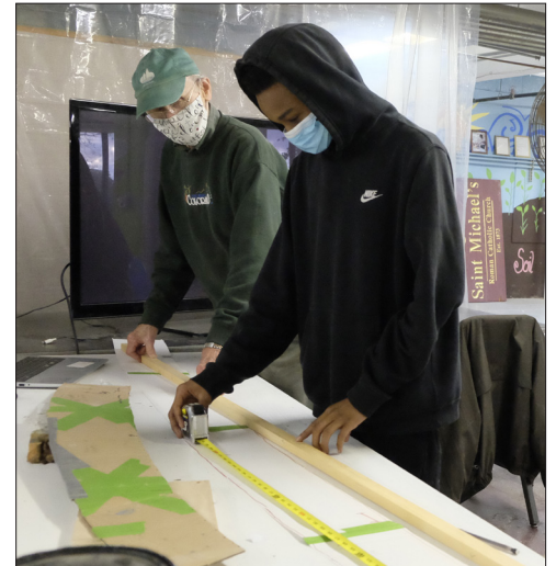
Jack Cargill and Yaqub measure the template for the curved top and bottom rails that will hold the shrine's wooden vertical struts in place behind the statue.
