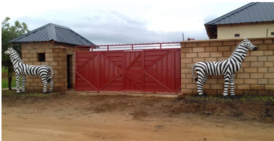
Guest house Entry Gate
