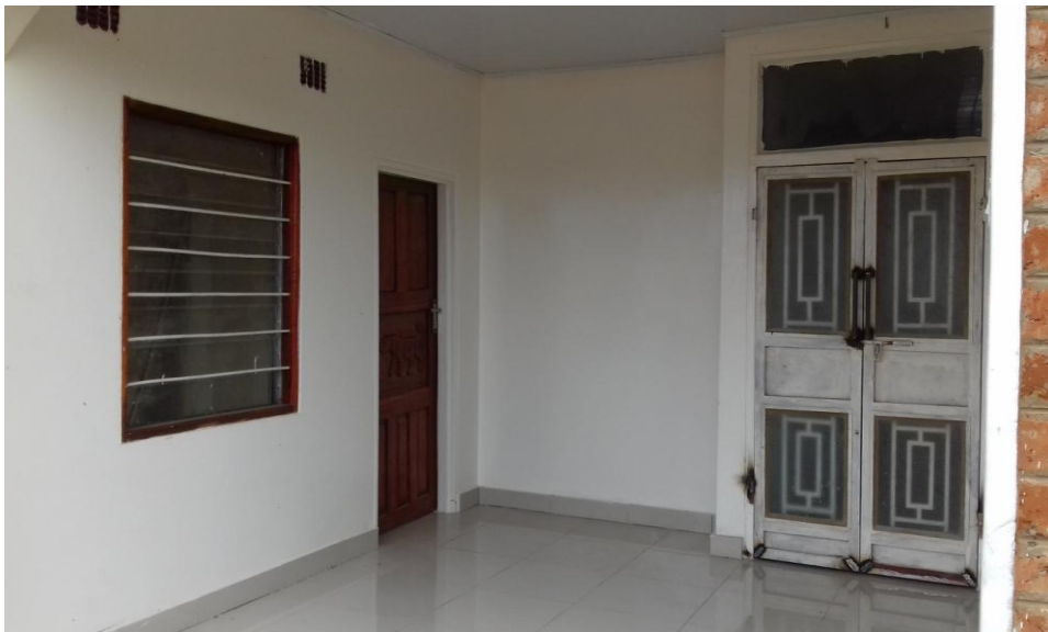
Tiles and glasses fixed
