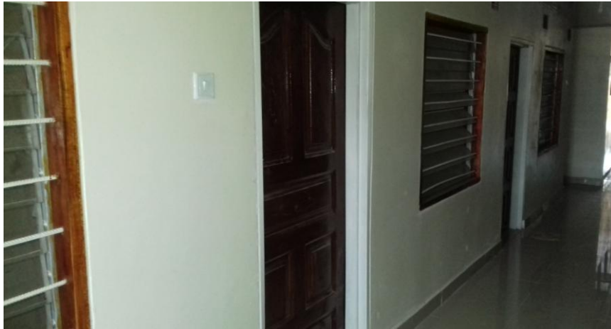
Guest rooms - passage view
