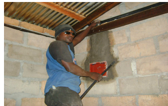
Canteen/Laundry plastering and wiring simultaneously in progress.
