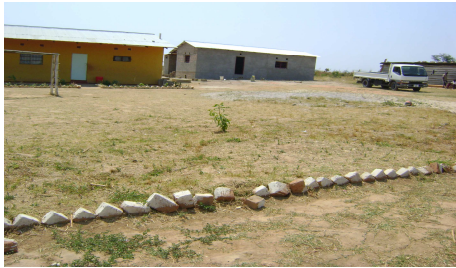
Surroundings continually clean
