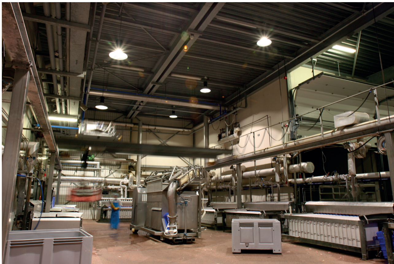
Cold storage room with LED High Bay 100 Watt and aluminium reflector.
