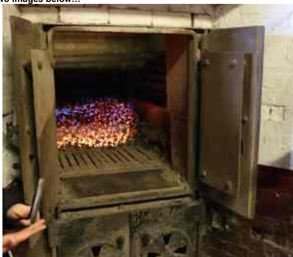
Anthracite (coal) being burned in the kiln at Balvenie. The coal gives off heat, but no smoke.
