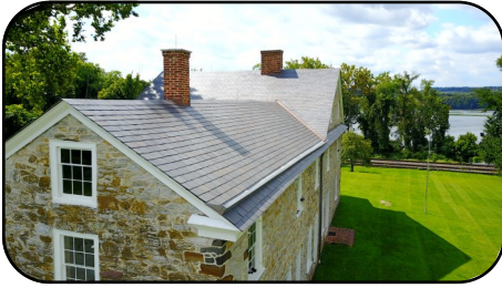
New Slate Roof Installed on Mansion, Chimney Masonry Repairs, Lightning Rods
