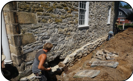
Mansion Foundation Masonry Repairs and Waterproofing
