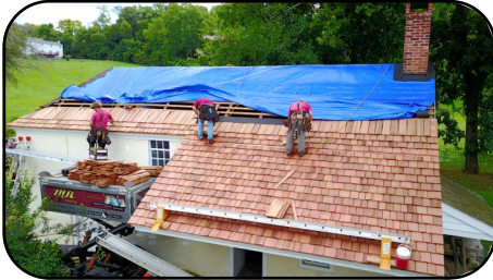
New Period Cedar Shake Roof Installed on Summer Kitchen
