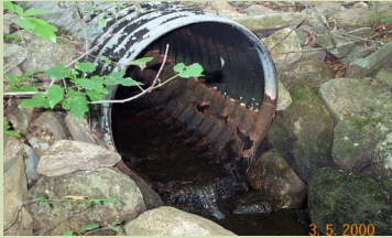
Perched Pipe Outlet—courtesy of CT DEEP
