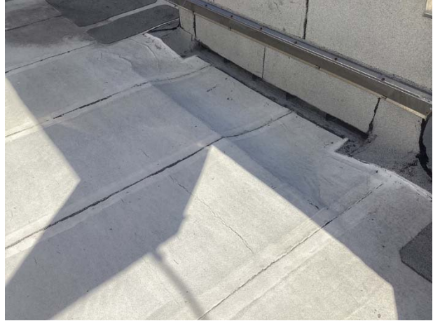
Coating cracks
