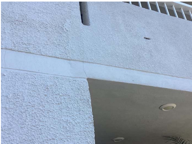
Stucco crack
