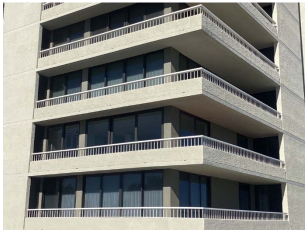
Aluminum railings overview
