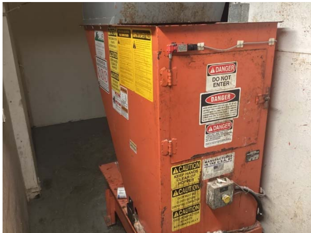
Trash compactor enclosure
