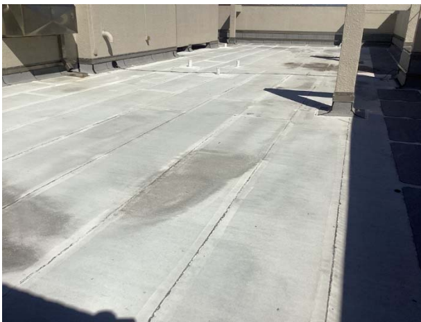
Modified bitumen roof overview
