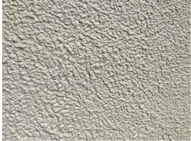
Typical stucco wall finishes
