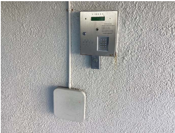
Access point at entrance
