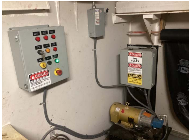
Trash compactor controls
