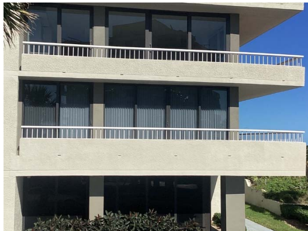
Typical aluminum railings
