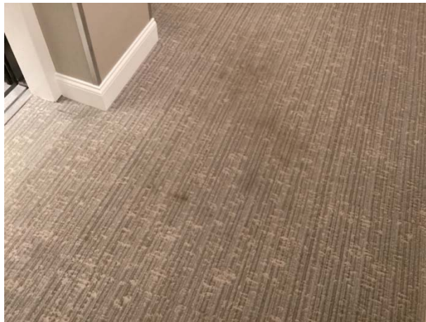
Carpet stains at floor 26
