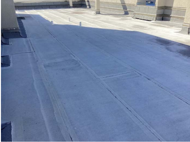
Modified bitumen roof overview
