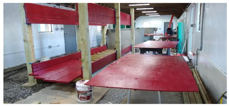
Progress on one of the two deep-water aquaculture growing beds. Behind the two growing beds are the tanks; not seen are the sediment filters, biofilters, and oxidation tank. In the front bottom of the picture is the platform for the vertical growing system.
