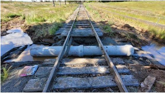
*Repairs underway to a culvert north of Borg's Gate 6. Photo shows the amount of water accumulating on either side of the track.*
