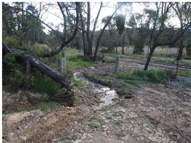
*Water flow off Black Bullock Road has been diverted into rail corridor and under the track to stop the new rail crossing from damage*
