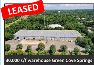
30,000 s/f warehouse Green Cove Springs
