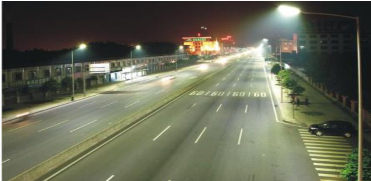
Figure 3.1 Typical project site
