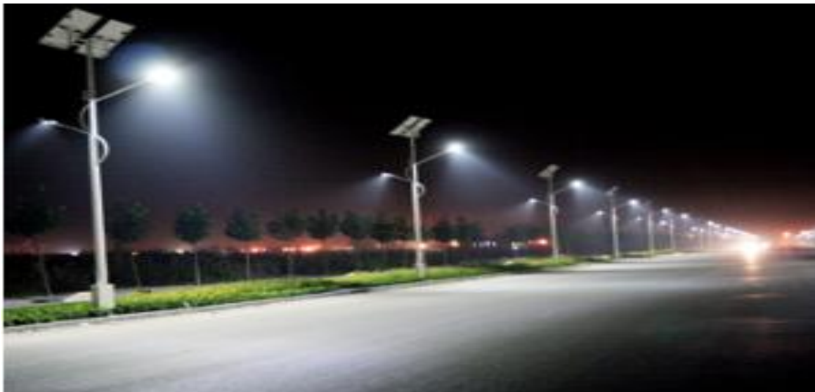
Figure 4.2 Example of PV solar street lights
