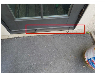
2.1 Item 2 (Picture) garage
