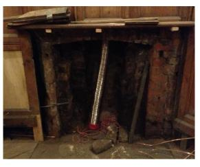
The story of the flue! As the work nears completion we see hidden aspects being put in place, for example the flue for the chimney, which will serve the new gas fire in the Rector's vestry. Once this is in place the Victorian fire grate and surrounds will be fitted.
