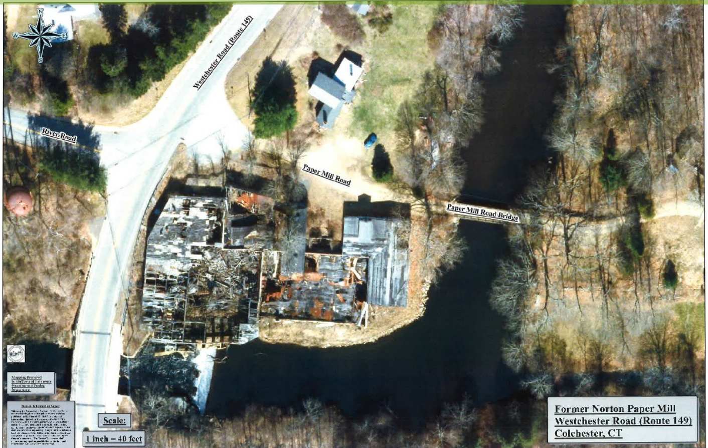
Aerial photograph showing top of the old mill. The dam is just south of the building, to the east of RT 149. Courtesy of J. Gigliotti, Town of Colchester
